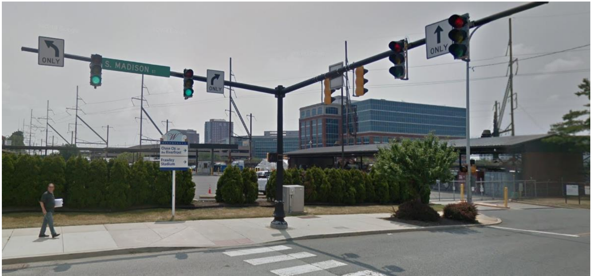
Read Street and S. Madison Street in Wilmington. The pole and mast arm are DelDOT's ornamental double mast-arm poles.
