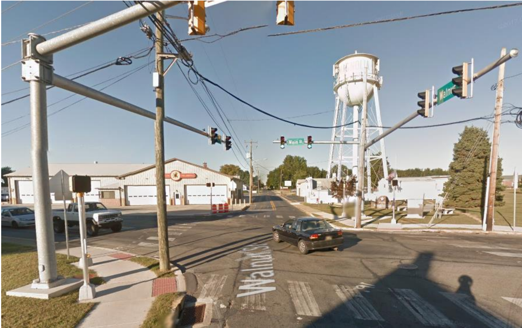
Main Street and Walnut Street in Magnolia. The pole and mast arm are DelDOT's standard double mast-arm poles.
