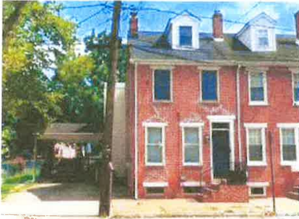
Flat roof section not visible from front [23 West 6 th St.]
