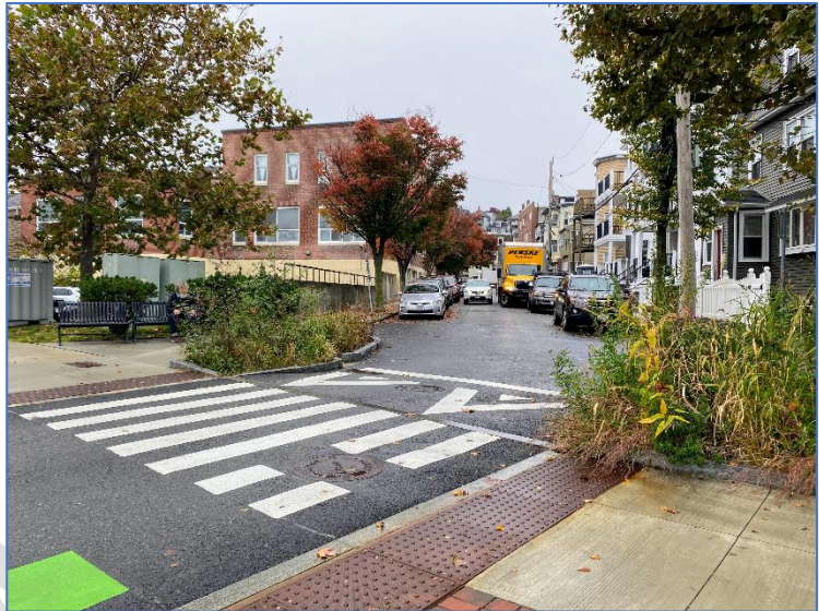
Curb bumpouts with landscaping and brickwork incorporated
