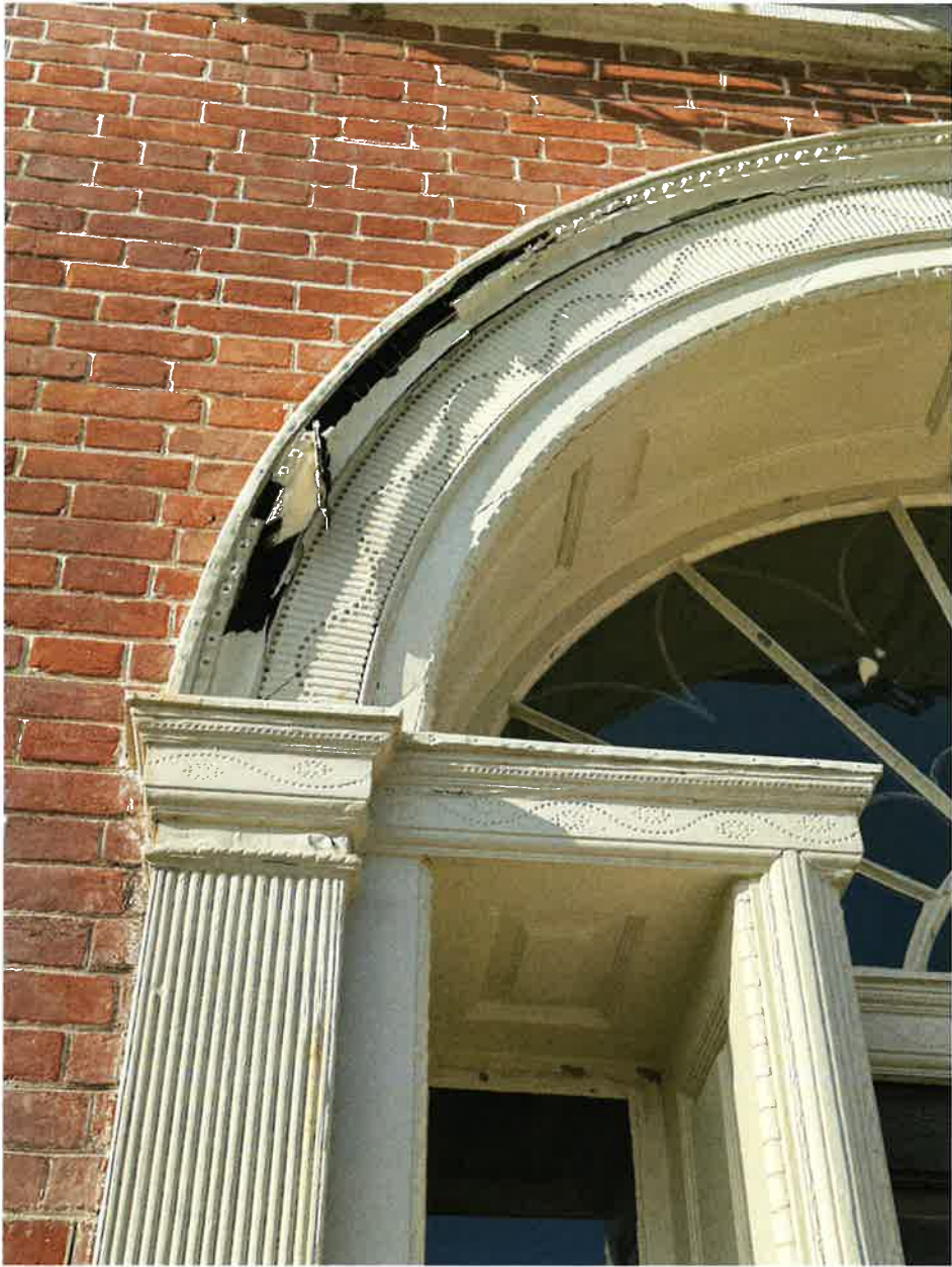
Close up of surface to be treated, taken December 18, 2025
