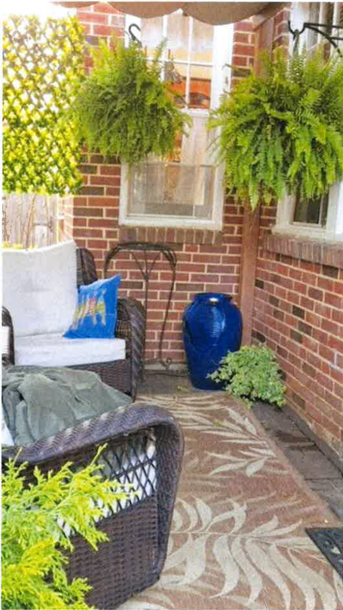
REPOINT AS NEEDED SIDE PATIO 1 st and 2 nd FLOOR EXTERIOR
