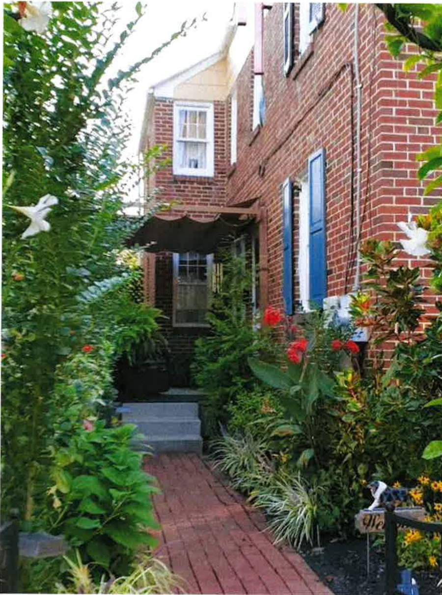
SECURITY LIGHT INSTALL ABOVE 2 nd STORY WINDOW
