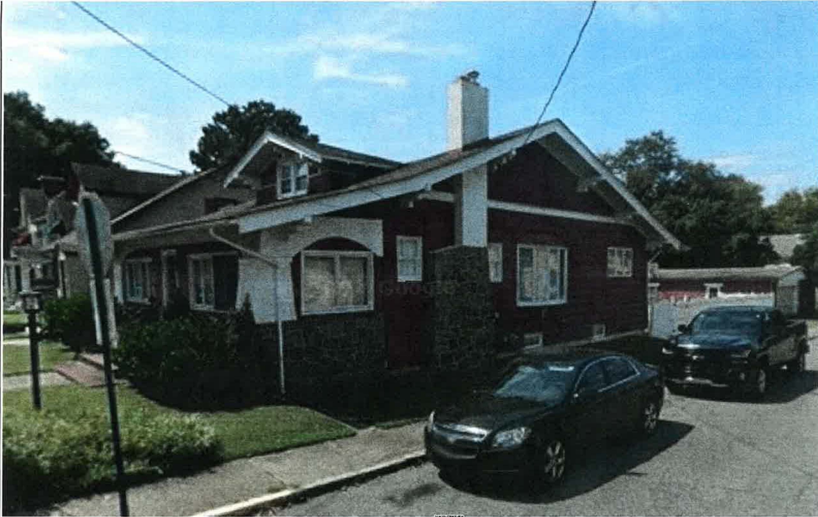
○ Corner View Existing House
